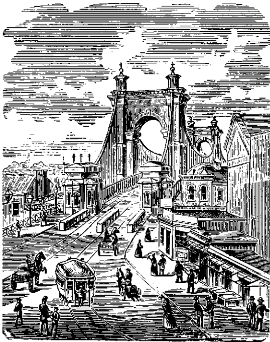
The Suspension Bridge.
